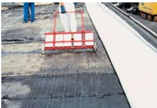
Pict. 1 Use of an applicator. When the adhesive is applied in lines, as illustrated, it must be squeegeed across the width of the membrane to create a full bond.
