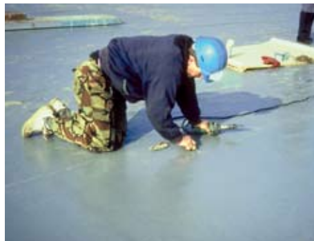
Fig. 2: Verification of weld security
