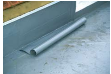
Fig. 3: Edge restraint with AlkorPlan® metalsheet 81170 or 81171
