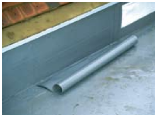
Fig. 3: Edge restraint with alkorPLUS® 81170 metalsheet
